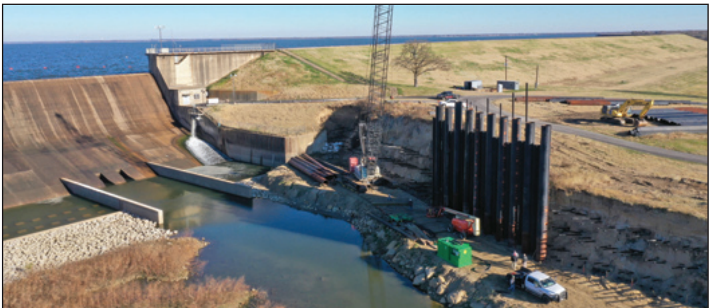
Lake Tawakoni Spillway Channel Bank Stabilization Project
