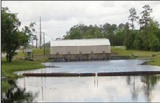
John W. Simmons Gulf Coast Canal Pump Station
