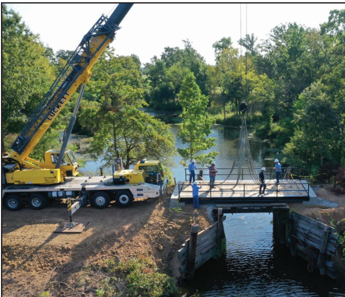
Caney Point Bridge Construction
