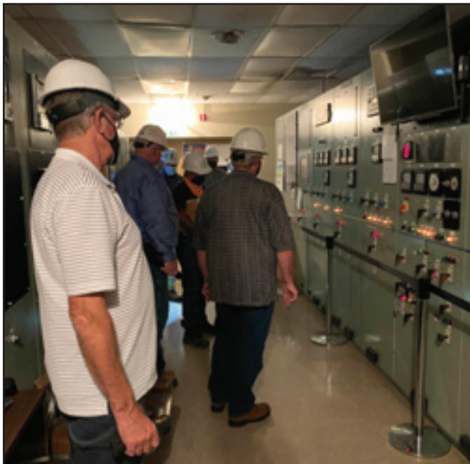
Toledo Bend Powerhouse Inspection
