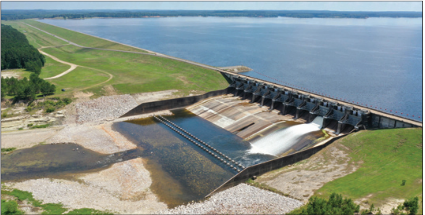
Toledo Bend Spillway Repair Completed
