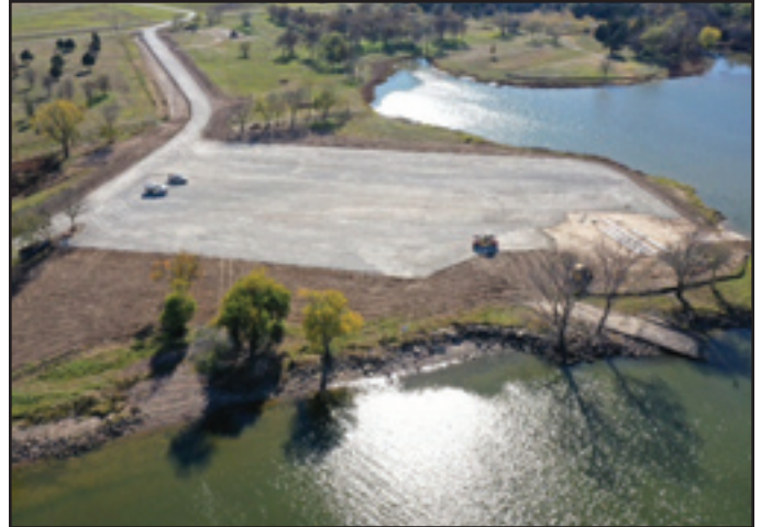
Construction of Additional Park Facilities
