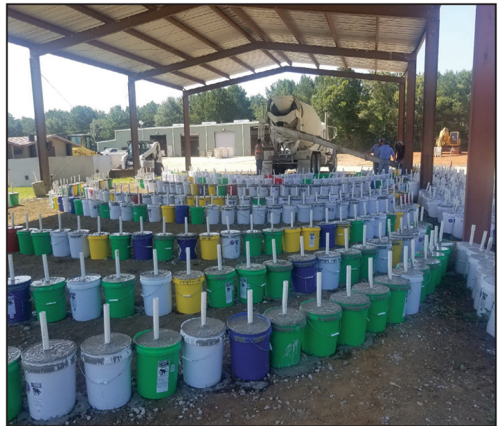
Assembling Buoy Anchors
