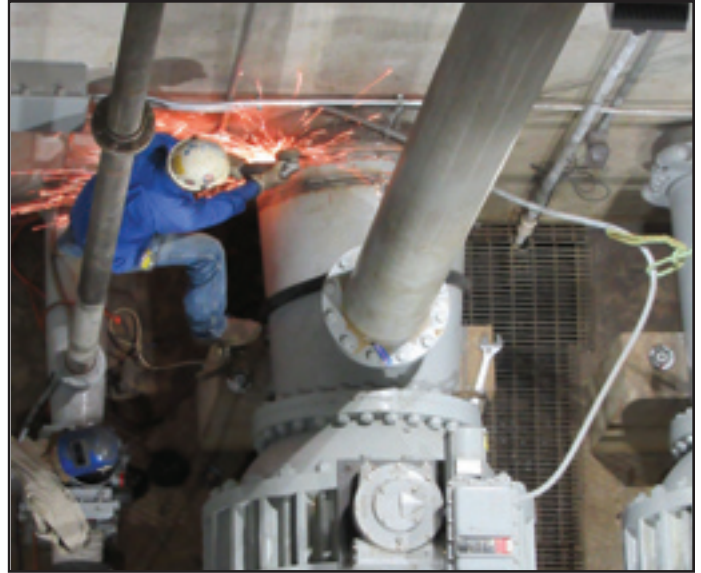
Lake Fork Dam Bypass 36-inch Pipe Maintenance
