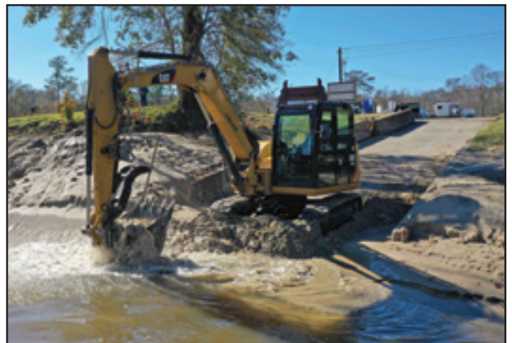
Clearing State Highway 12 Sabine River Boat Ramp
