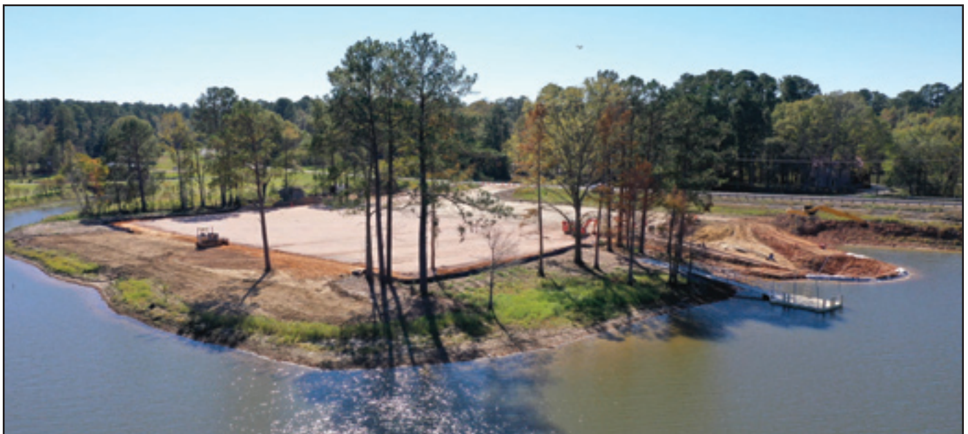
Six Mile Boat Ramp Facility Improvements
