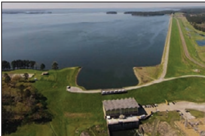
Toledo Bend Dam and Reservoir
