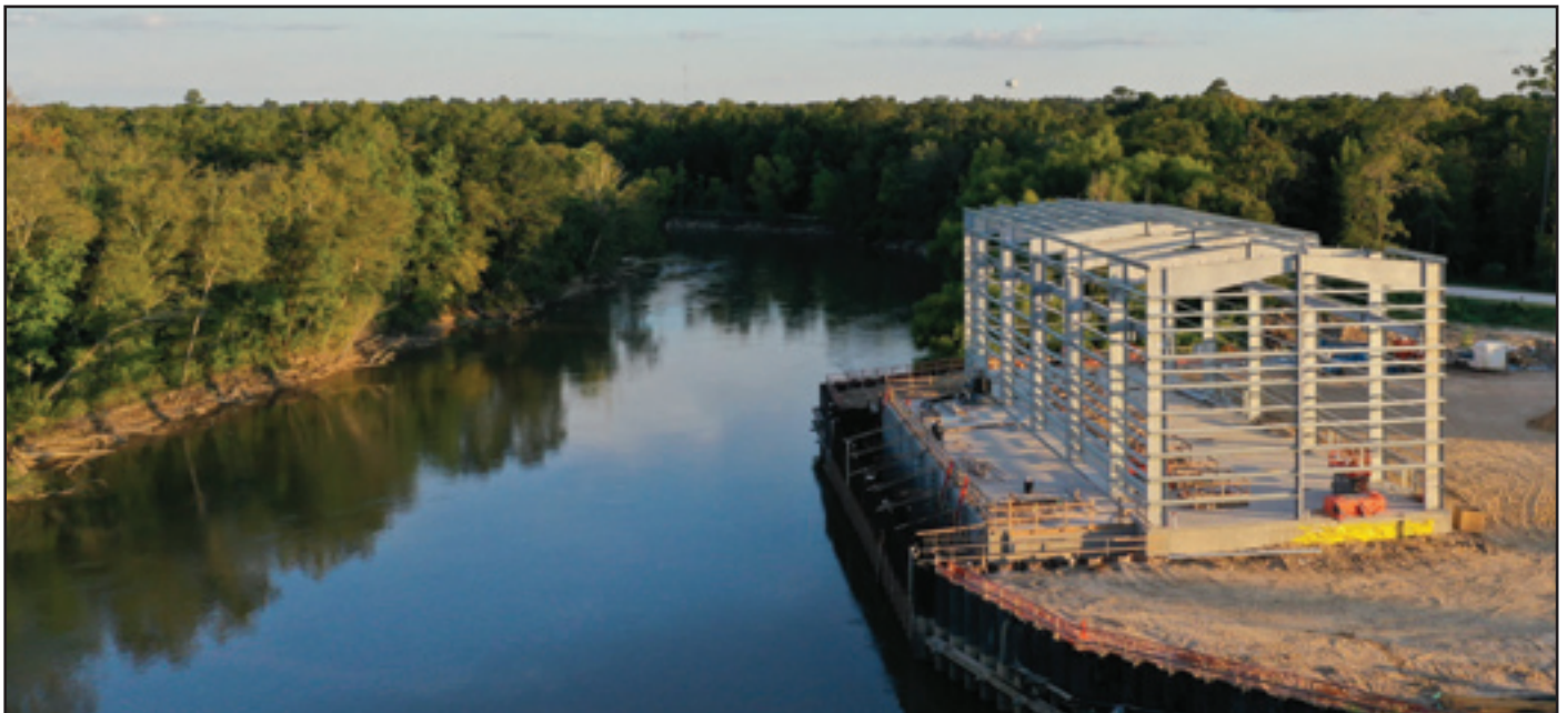
Ongoing Construction of New Pump Station off State Highway 12
