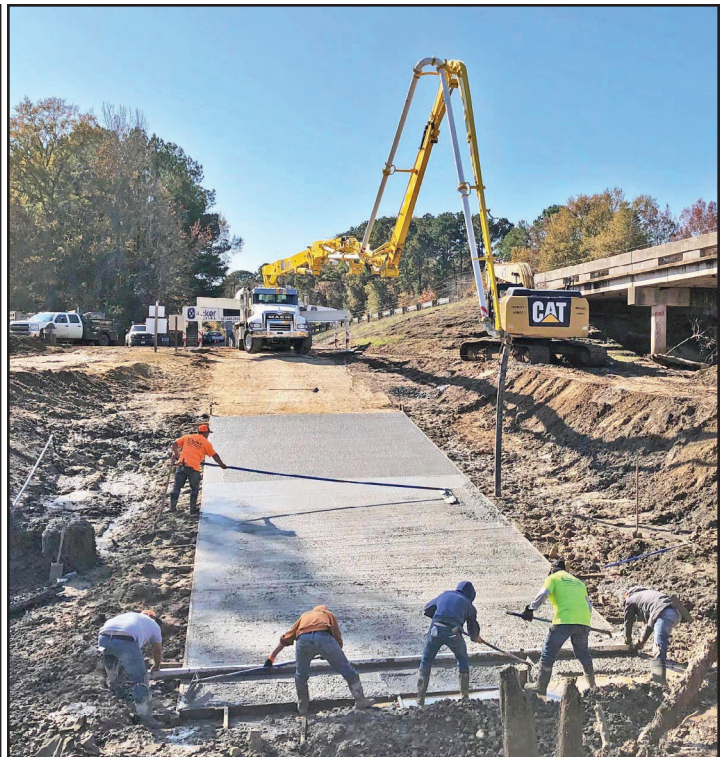
Bubba Cowser Boat Ramp Repairs and Extension
