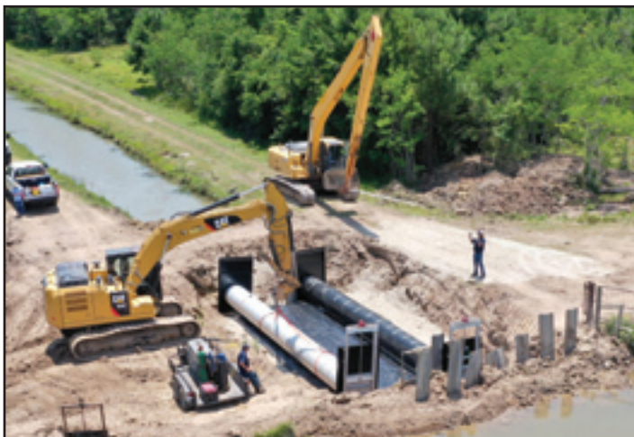
Constructing New Control Gate at Allied Check
