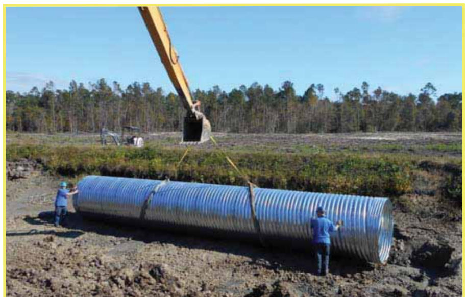
Installation of New Road Crossing Culvert
