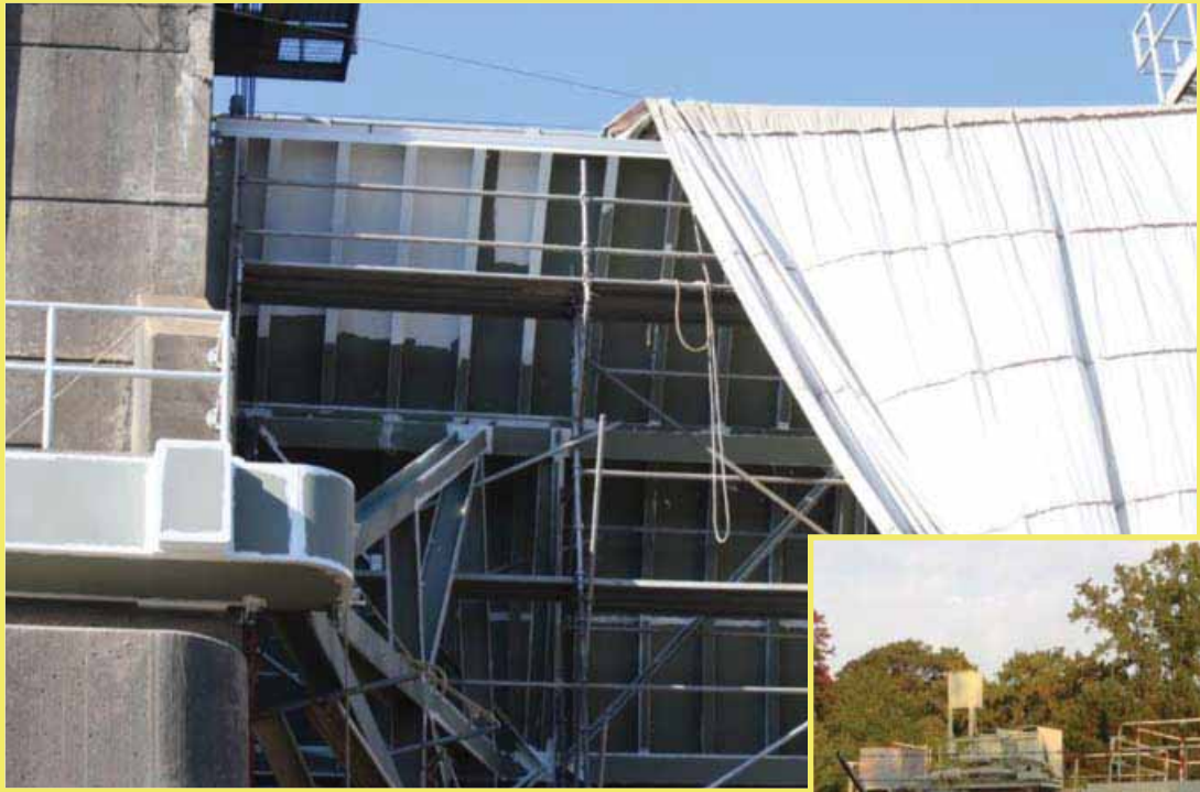
Gate Refurbishment at Toledo Bend Spillway
