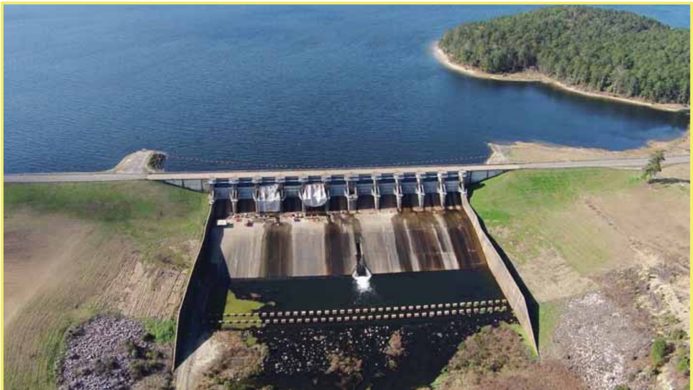
Gate Refurbishment at Toledo Bend Spillway
