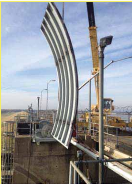
Tainter Gate Face Plate Section Installation
