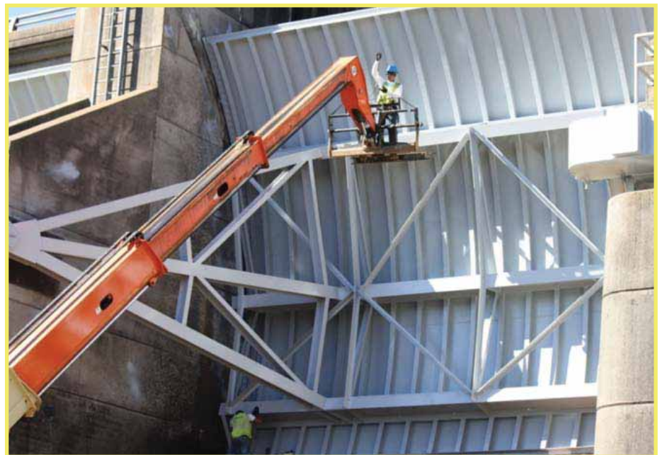
Newly Refurbished Spillway Gate at the Toledo Bend Project
