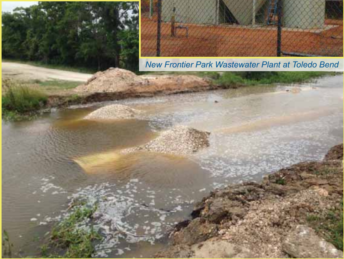
Replacing Road Crossing in GCD Canal
