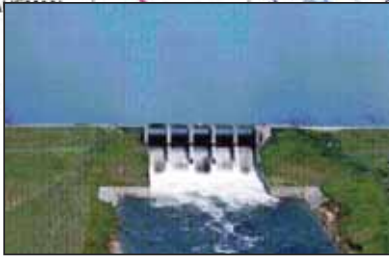
Lake Fork Dam & Reservoir (1980)
