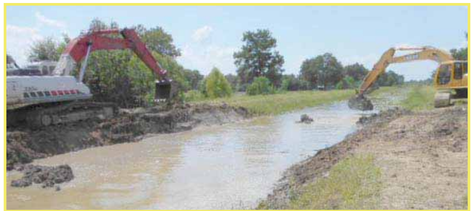
Canal Levee Maintenance
